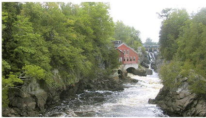
low-impact hydro projects
